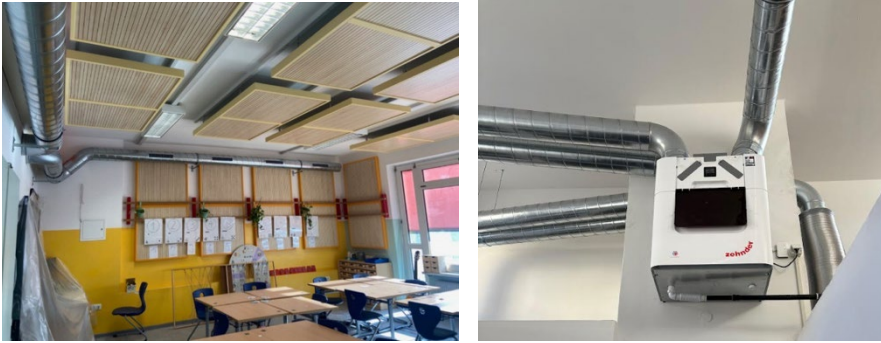
Figure 1. Distribution system in the classroom (left) and VMC installed in the bathroom (right). One machine dedicated to each classroom. Primary school in Bolzano.
