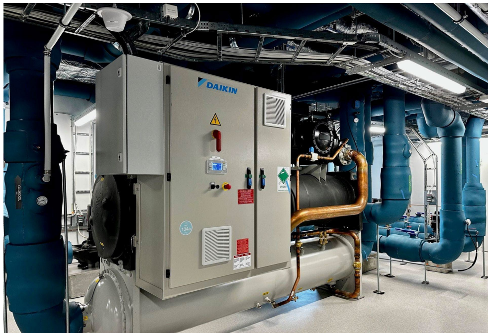
Fig. 5. Picture for illustrative purpose (non-exhaustive) from Daikin Applied Europe S.p.A. of High Temperature HP Water to Water EWWH- VZ with nominal heating capacity (depending on the size and features selected) from 400 – 1900 kW, using low GWP Refrigerant, R-1234ze, with Inverter driven Screw Compressor. It can be suitable for being used in several applications of waste heat recovery. With “modular combination” they can scale from 2 to 10 MW and more of heating capacity with stable and reliable technology [19]
