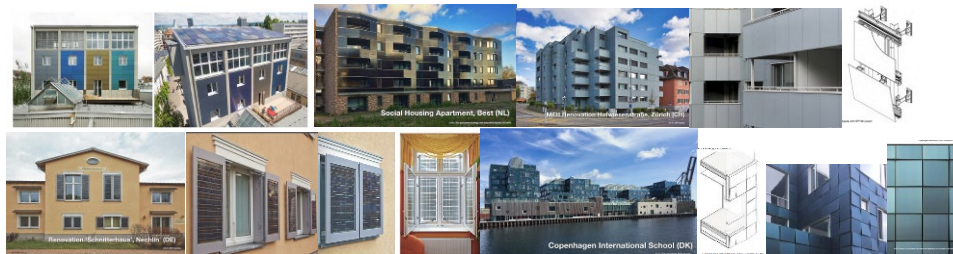
Fig. 2. First two images represent colourful printed custom-size solar panels for facades applying SissINSO Kromatix™ – Solar Silo Kahlesio, Basel (CH), Industrial buildings (from SUPSI; http://www.bipv.ch ). Other images are projects taken from [21]
