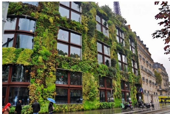
Fig. 3. Vertical landscaping of facades of Patrick Blanc.
