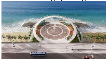
Figure 7. Overall perspective of the multifunctional breakwater.
