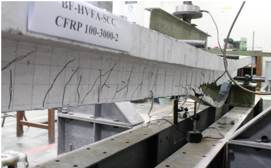
Fig. 8. Crack Pattern on Test Beam Specimen with CFRP Strengthening (BF-HVFA-SCC-CFRP100-3000-2)
