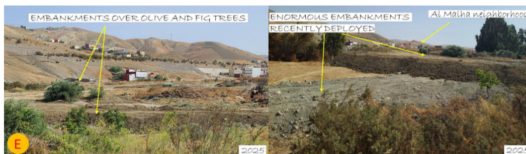
Fig. 8. Construction debris deposited over fruit trees in the floodplain at section E.
