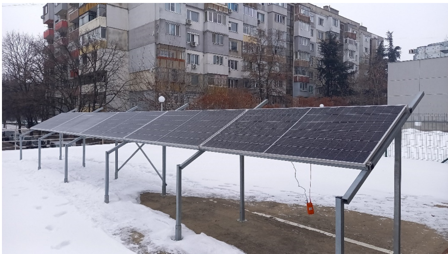
Fig. 1. Bifacial PV string on the campus of the University of Ruse.
