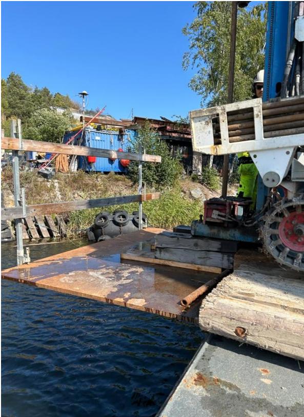
Fig. 4. Site investigations along the shore from a barge.
