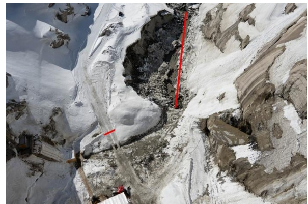
Fig.12. Collapse of lacustrine sediments following depressurization of the diversion tunnel. The vertical red line indicates the main collapse axis and direction of sediment displacement, while the dashed line indicates the approximate extent of the failed mass.
