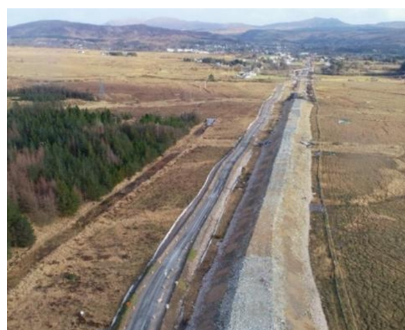
Fig. 1. Temporary diversion on left and main embankment at surcharge level.
