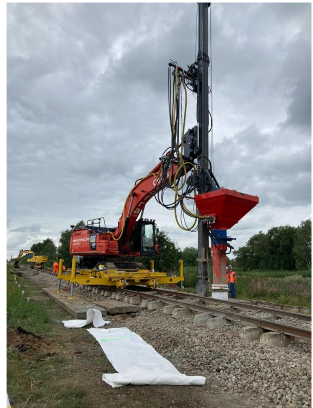
Fig. 7. Installation of gravel columns under embankment and track.
