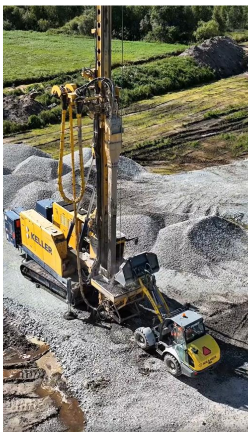
Fig. 3. Installation of stone columns – Harju 2 site.
