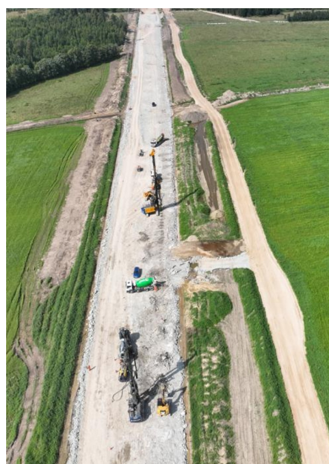
Fig. 4. Installation of rigid inclusions –Rapla 4 site.
