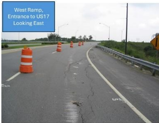
Fig. 5. West ramp pavement cracks in 2004.
