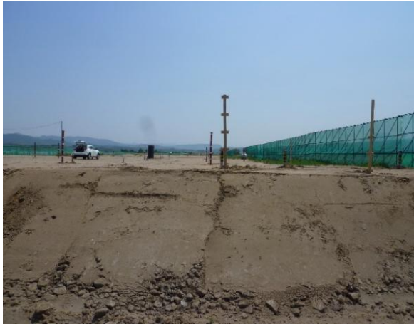
Fig. 4. Embankment construction status.
