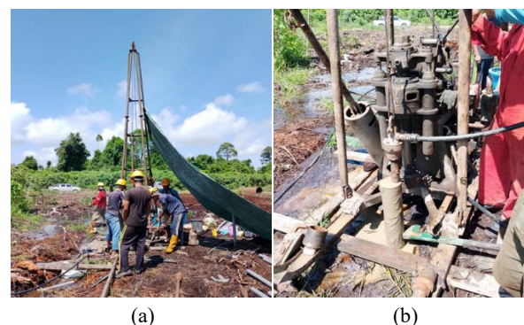
Fig. 2. Boreholes drilling: (a) setting up of SI drilling machine, and (b) drilling works.
