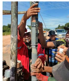
Fig. 7. Installation of spider magnet extensometer.
