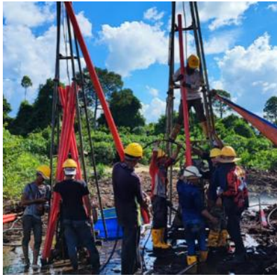
Fig. 3. Installation of inclinometer.
