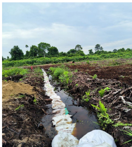
Fig. 8. A cable trench was dug to lay cables below embankment construction and covered with sandbags as protection.
