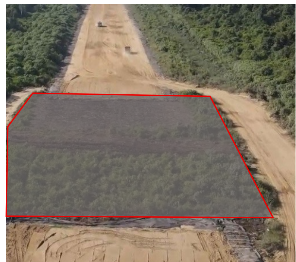
Fig. 2. Study area during road construction.
